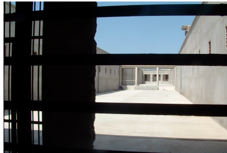
One of the courtyards of the new prison that is being built in San Martinho, near Praia, Santiago Island. November 2008.
