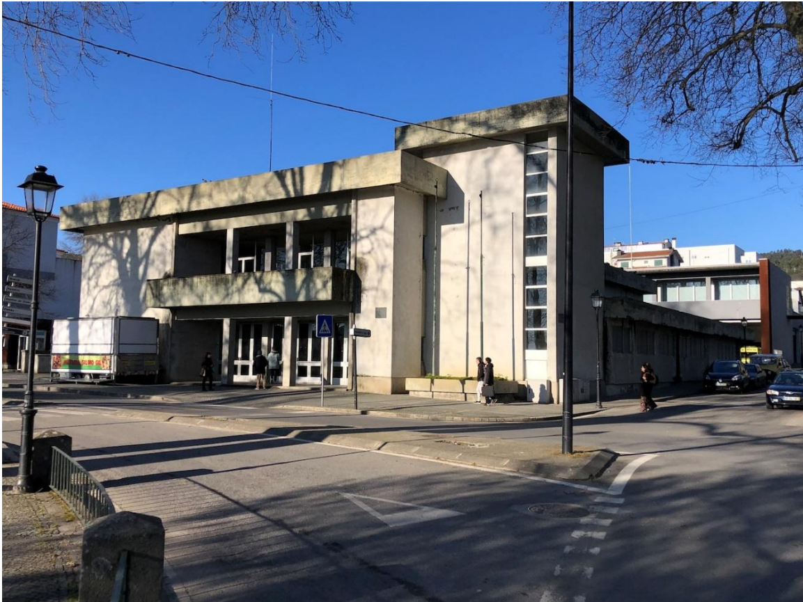
FIGURE 1. FIRE BRIGADE STATION IN ALIJÓ, 2023
